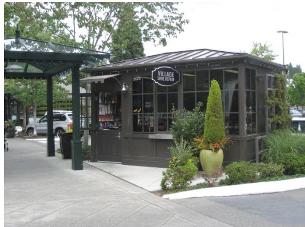
Specialty building or kiosk.
