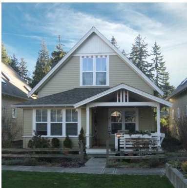
Entries including door, windows and porch, should be given special attention.
