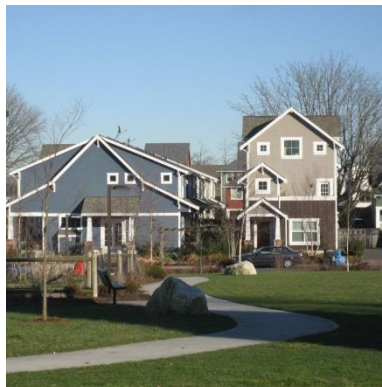
A variety of roof forms adds interest to a neighborhood.
