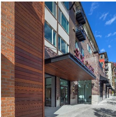
Enhanced main entry
